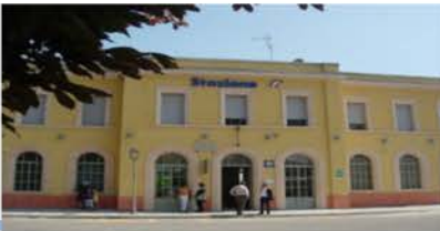
Rail Infrastructures and Services: Connect
