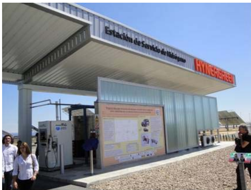
Figure 3.56. Hydrogen fueling station. (Source: Hércules Project)
