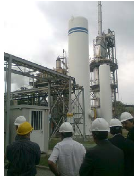
SOL plant in Ravenna
